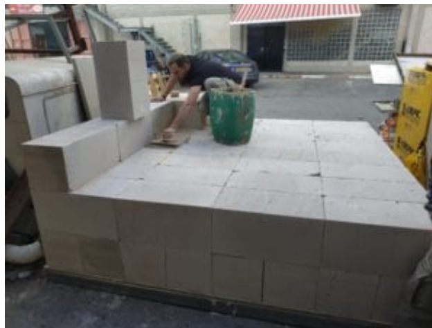
Constructing the altar (courtesy: Sanhedrin)
